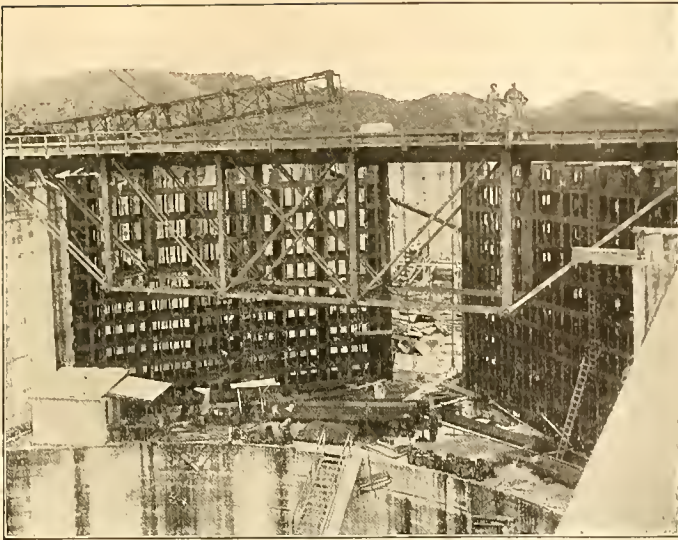
BUILDING AN UPPER TIER OF LOCKS
